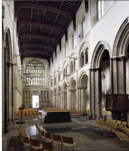
Rochester Cathedral Nave Photo C. Jilks
